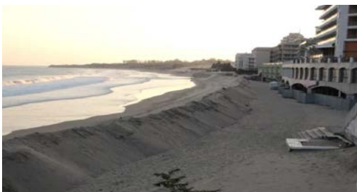
Fig. 4. Recent development in the New town of Nesebar: (a) densification and resulting silhouette; (b) damages on the beach
