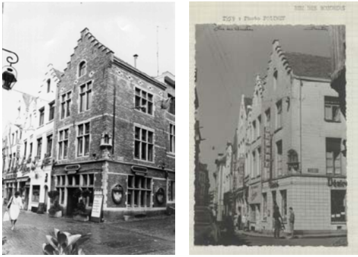
Fig. 7 Rue des Bouchers, before (1959) and after (1980) works
