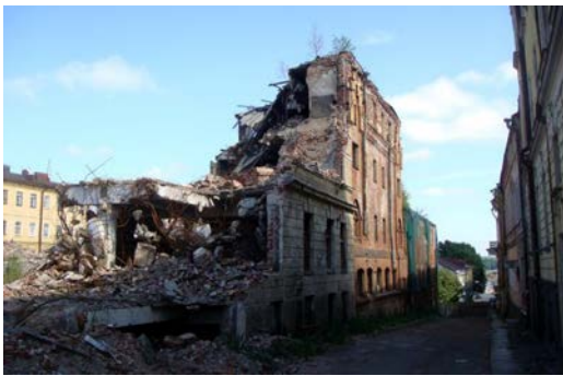
Fig. 7 The ruins of the urban quarter delimited by the streets Krepostnaya, Krasnoarmeyskaya, Storozhevoy Bashni, and Krasina, in 2013. There are places in the town where it seems as though it was only yesterday that the war ended. The city-owned block that was almost completely demolished in 2013. Photo Netta Böök
