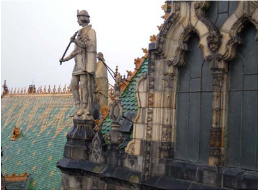
Fig. 1 Details of a historic building from the end of the 19 th century
