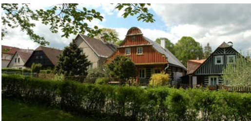
Fig. 14 The heritage reservation protecting the ensemble of vernacular architecture inside a little East-Bohemian town of Lomnice nad Popelkou (quarter Karlov) (Karel Kuča 2008)
