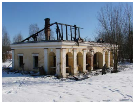
Fig. 9 Guardhouse in the Annenkronne fortress, damaged in a fire, viewed in 2013. Photo Netta Böök
