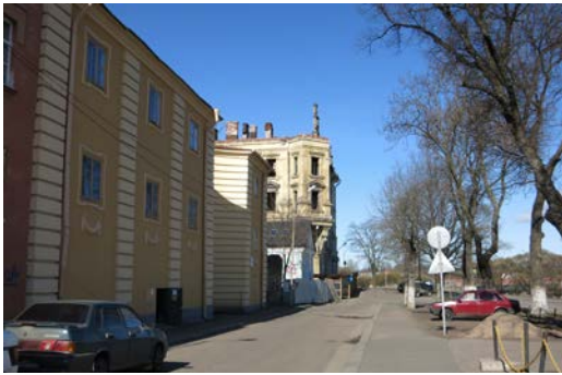
Fig. 6 In July 2014 a fire destroyed the roof, corner tower and two upper storeys of the Neorenaissance building at Severnyi Val 11 dating from 1897. In June 2016 the building was still unprotected from rain and snow. Photo Netta Böök
